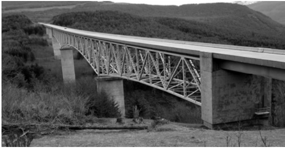
Figure 2 Bridge crossing a valley
