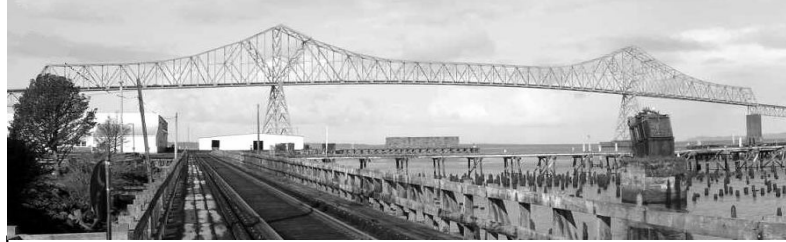
Figure 1 Bridge crossing a river and a railway yard.
